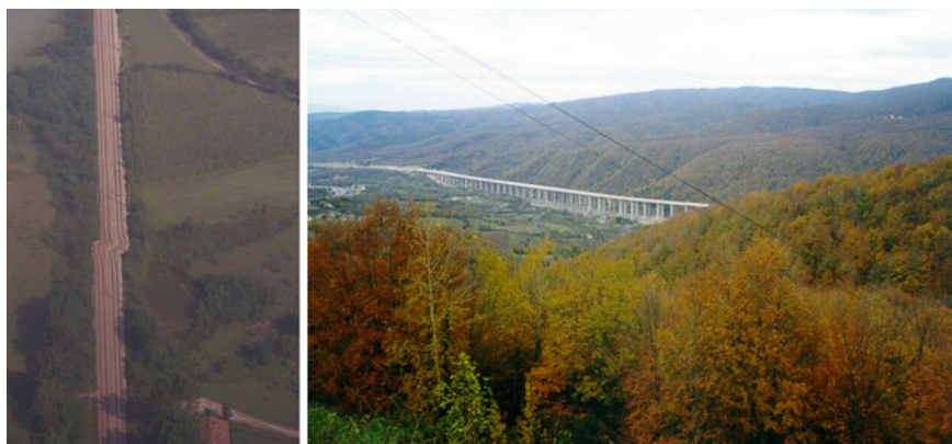
Fig. 1.33 Fault rupture crossing a railway track ( left ) and a viaduct ( right )
