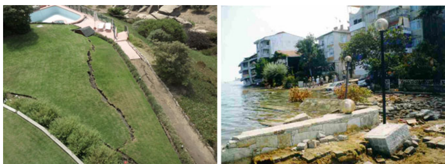
Fig. 1.37 Lateral spreading in the Olas development landscaping during the 2010 Maule, Chile earthquake ( left panel EERI Earthquake Photo Gallery) and buildings dragged into the sea due to lateral spreading in Gölcük during the 1999 Marmara earthquake ( right panel )
