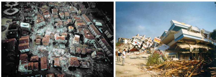
Fig. 1.32 Left Uneven distribution of damage in buildings located in the same area, subjected to the same ground motion. Right Totally collapsed buildings, which killed their occupants
