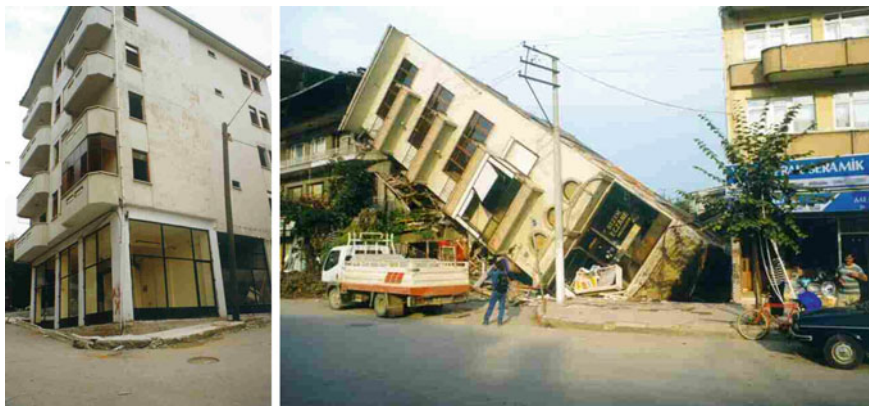
Fig. 1.36 Tilted buildings on liquefied soils in Adapazarı during the 1999 Marmara earthquake
