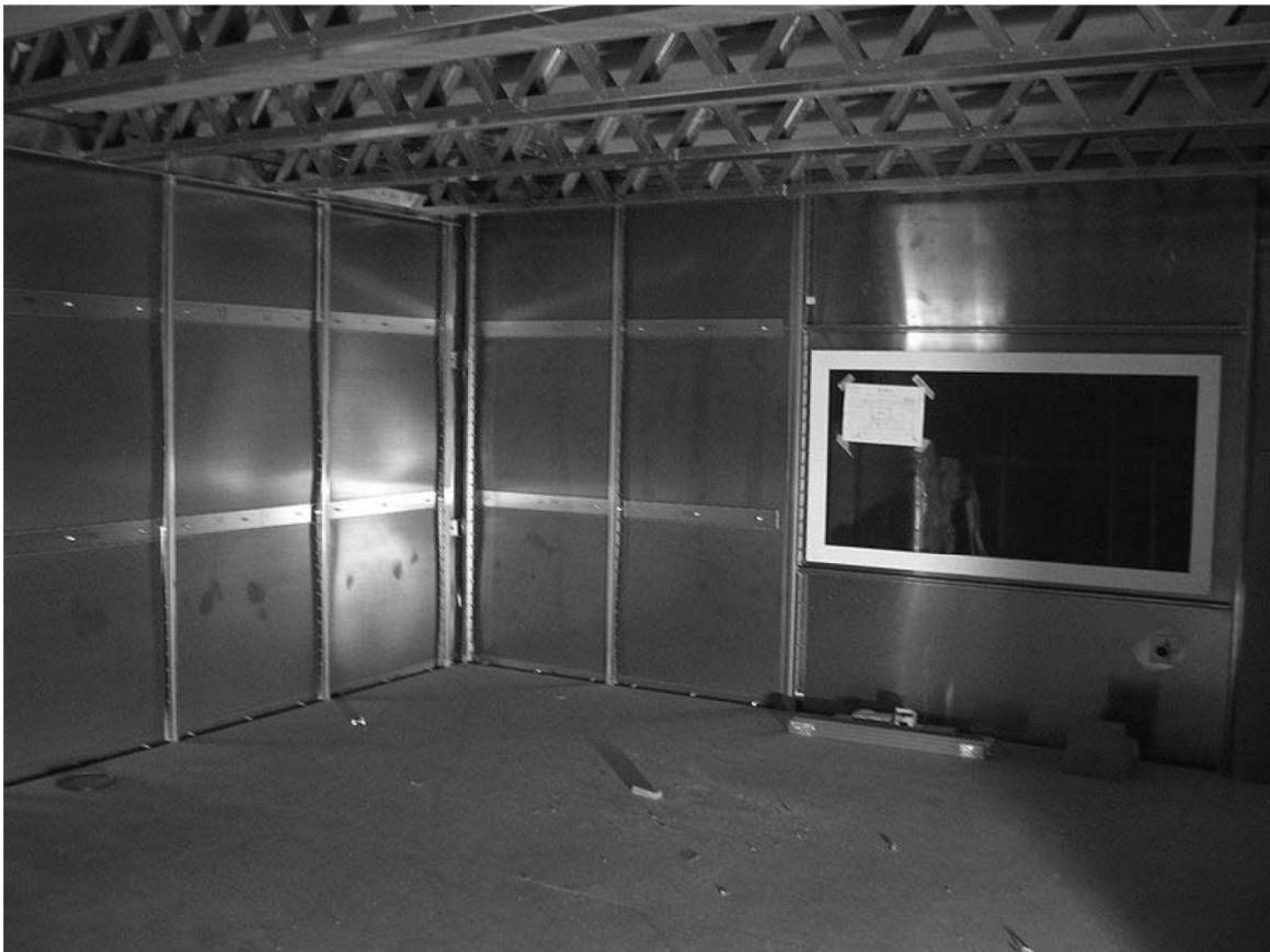
Figure 2.17: An example Faraday cage. (Image by M. Junghans; licenced under the terms of the GNU Free Documentation License, Version 1.2.)
